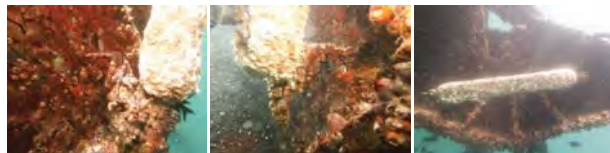
03 #5 Chain Stopper Anode Left (4)
